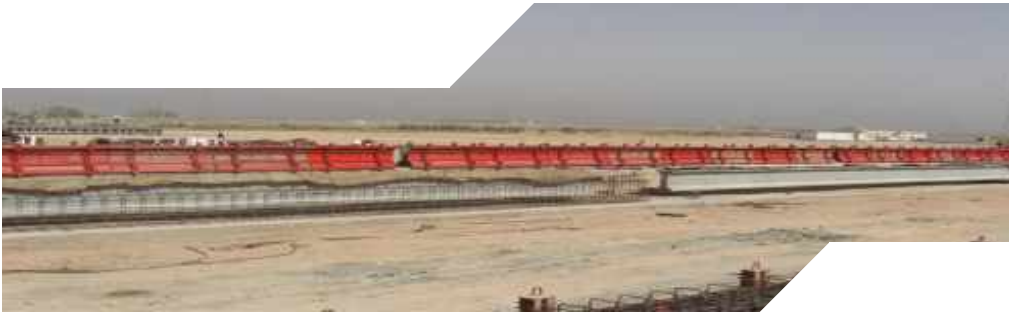
Al Shamiya Bridge, Iraq
