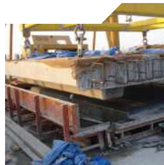
Slab & Beam Moulds
