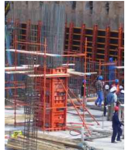
Tripoli Tower, Libya
