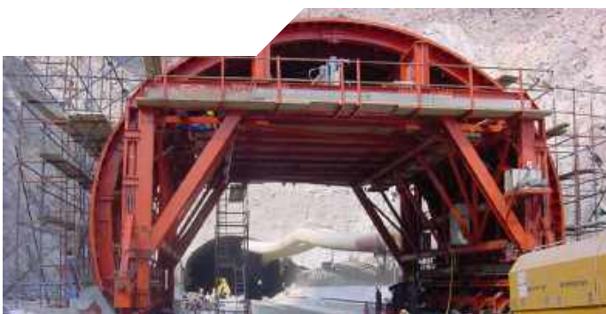
Wadi Muddiq to Gillay Tunnel, UAE
