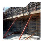
Modular components Reduces time to assemble and dismantle panels.
