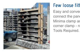
Few loose fittings Easy and convenient to connect the panels by using Minima clamp and Minima corner clamp - no Special
