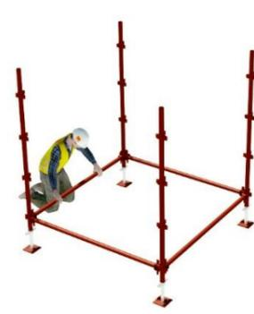
The operatives each prepare another leg (standard and base) and connect these to the free ends of ledgers protruding from the initial frame.
