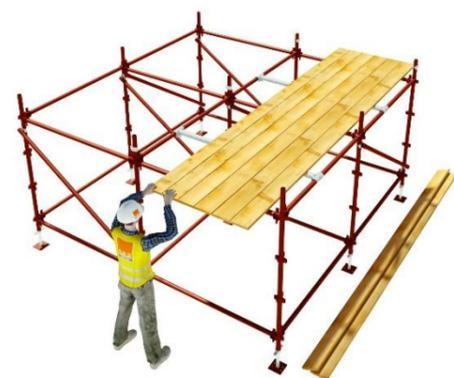
Once the bottom lift is complete, place scaffold boards/steel hook on boards on the top ledgers (using intermediate board supports where required) to provide a platform to erect the next level of standards.
