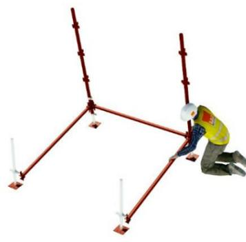
The operatives lean the constructed frame inwards and, whilst holding it with one hand, attach ledgers into the first set of pressings at the bottom of the standard. The frame is now self-supporting.
