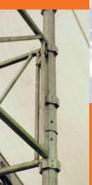
visibly safe and quick connection, allowing the frame to be installed or removed
